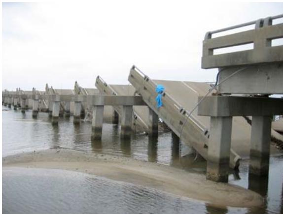
**Figure 1. US-90 bridge from Bay St. Louis to Pass Christian showing dislocation due to buoyancy and hydrodynamic loads [4]**
