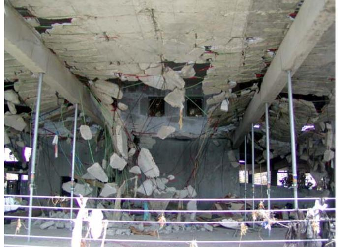
**Figure 2. Parking garage post-tensioned flat slab destroyed by hydrodynamic uplift forces. Note concrete shear wall and ramp obstructing flow through the building [5]**
