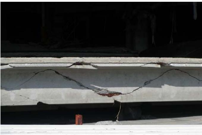
**Figure 1. Double-tee negative bending failure in parking structure at Grand Casino, Biloxi – bottom picture is inset from top picture [5]**
