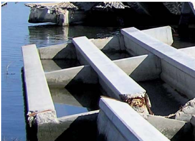
Figure 2. Inverted deck showing potential trapped air volume.
