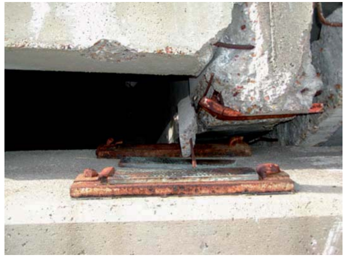
Figure 3. Friction bearing supporting US90 bridge girders.
