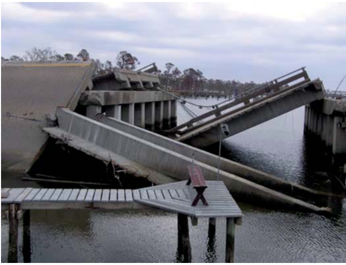
Figure 4. Deck segments of US90 bridge at St. Louis Bay.
