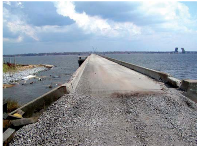
Figure 17. Railroad bridge over Biloxi Bay, Mississippi.
