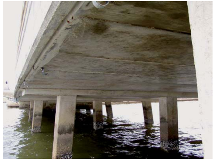
Figure 16. Undamaged bridge deck cast integral with support piles.
